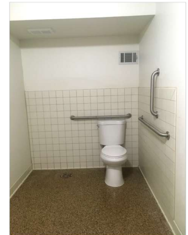
Outdated and unsanitary restroom surfaces were replaced with sanitizable tile and accessibility features were added.
