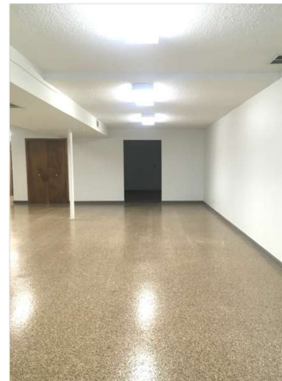
The basement carpet was replaced with an epoxy floor covering for better hygiene and durability. Walls were refreshed with new paint, and fluorescent lighting was replaced with LED for better collection care.
