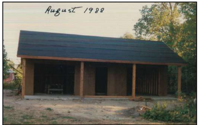
Carriage House during Construction. 1988. PHS Collection
